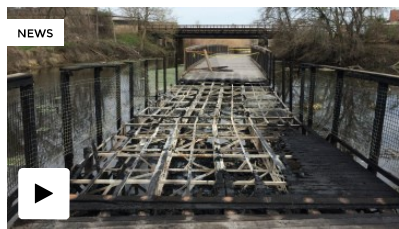
Towpath bridge in Akron destroyed by arson
